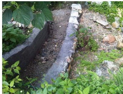
“Box drain requiring repairs”
